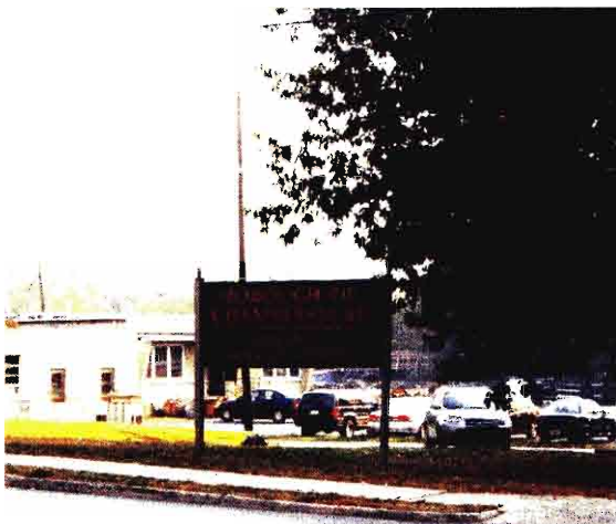
Utilities Service Center on S. Franklin St.
