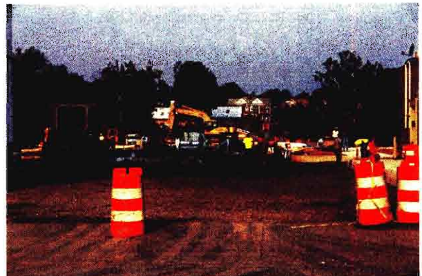
New Rosedale Parking Lot under construction
