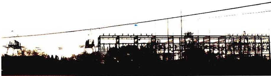
The expanded Cree Electric Substation on Walker Road
