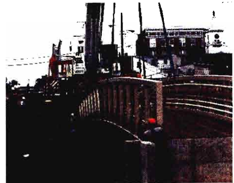
New footbridge over the Conococheague Creek
