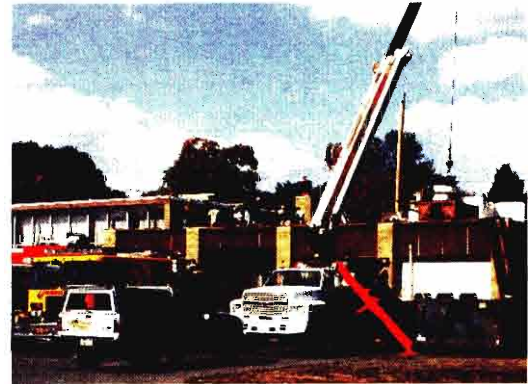
New roofs installed on the McKinley Street Fire Station
