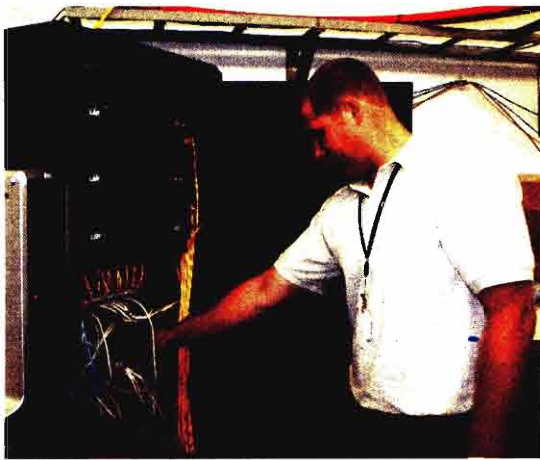
IT Tech Shawn Chilcote checks phone equipment in Borough Hall
