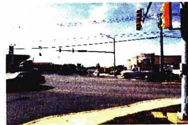
Additional lane on Orchard Drive at Wayne Avenue
