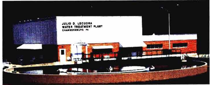
Clarifier at the Water Treatment Plant
