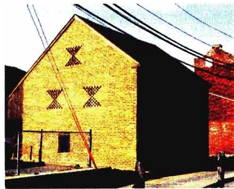
Restoration Project in downtown
